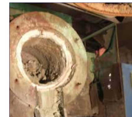
Ready to push out with the hydraulic push out system
