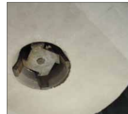
Lifting device without steel bottom plate
